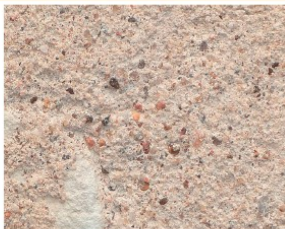
Grand-Pressigny - four banal - finition talochée
